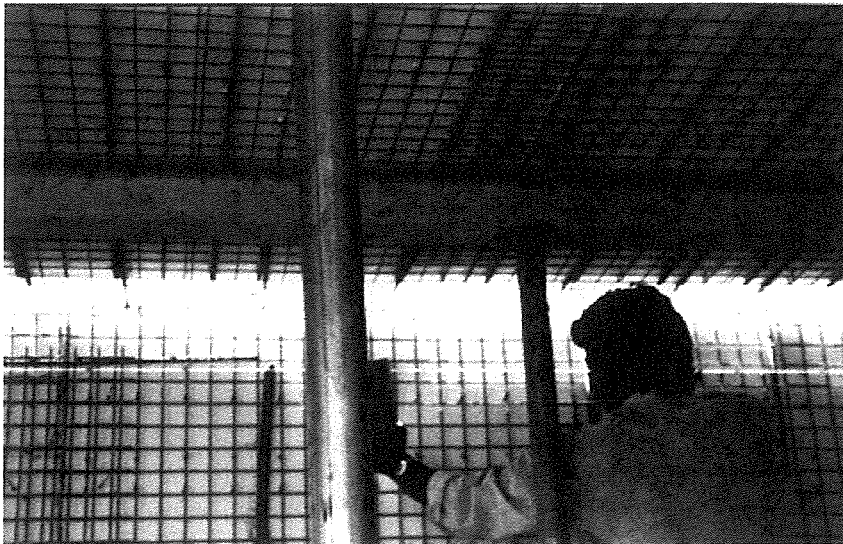
photo 6: Aligning the wall with a cord
