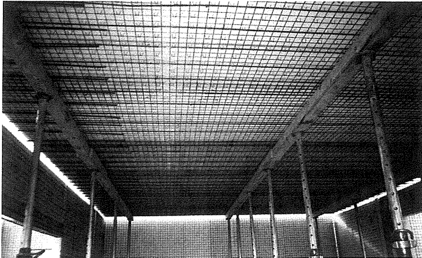
photo 7: Shoring the slab
