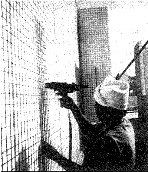
photo 3: Fixing of splice mesh with a hogging gun
